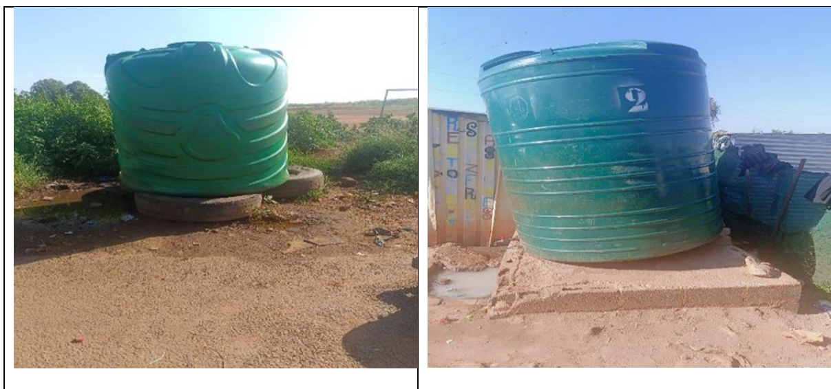
Figure 16a and 16b: Tank 8 sitting on low position. Source: Researcher (2024) and Lifted tank 7. Source: Researcher (2024)
