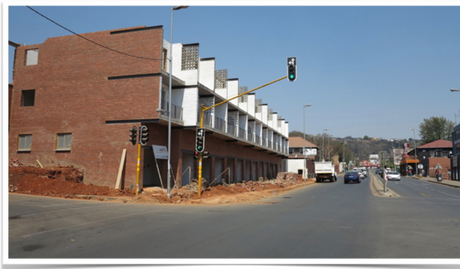
Figure 7: A new building project on Louis Botha Avenue, small shops on the ground floor with apartments on the first and second floors.
