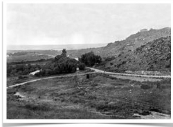
Figure 2: View of the original Louis Botha Avenue
