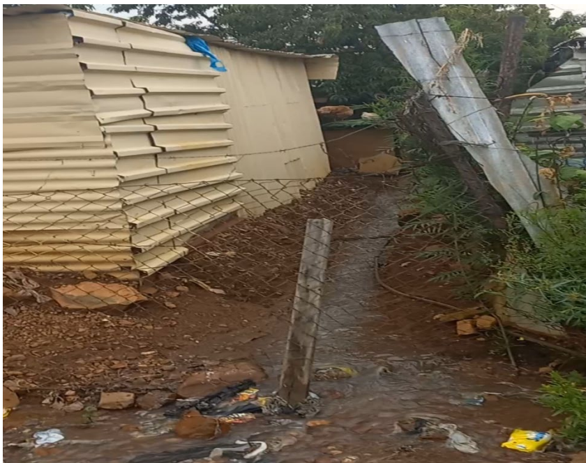
Figure 14: A picture showing sewage flowing from the bucket toilet all the way to the streets (picture by researcher)
